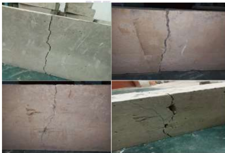
Figure 26: Failure of specimens
